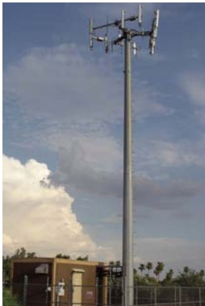
Fig. 1 A typical base station antenna and installation. ▼
